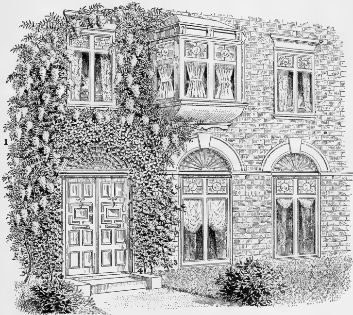
Fig. 75. CLIMBERS AND BLANK WALLS.
